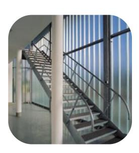
High daylight influx combined with restricted transparency and a functional/industrial aesthetic were decisive factors in using Pilkington **Profilit** or the building's façade.
