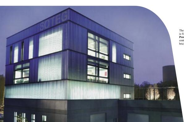
The workshop building's façade is fitted throughout with Pilkington **Profilit"**, which provides a stark contrast to the redeveloped brick buildings.
